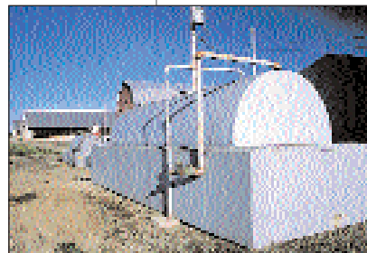
To store petroleum products safely, managers of Table Rock Farm, Castile, N.Y., use a concrete "bunker" around the tank.
